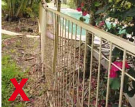
A fence in disrepair can lower the height of the barrier or provide a gap for a child to enter the pool area.
