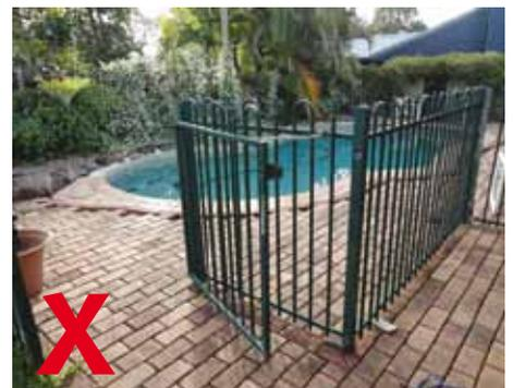
A gate cannot be tied or propped open and must self-close from any position.
