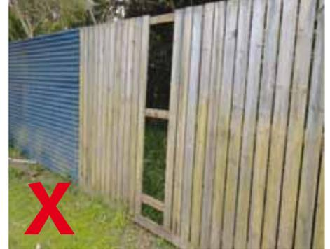
Gaps in a fence over 100 millimetres can provide easy access to the pool area.
